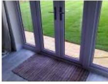
The FD is showing a significant issue with cold air ingress along the foot of the door.
